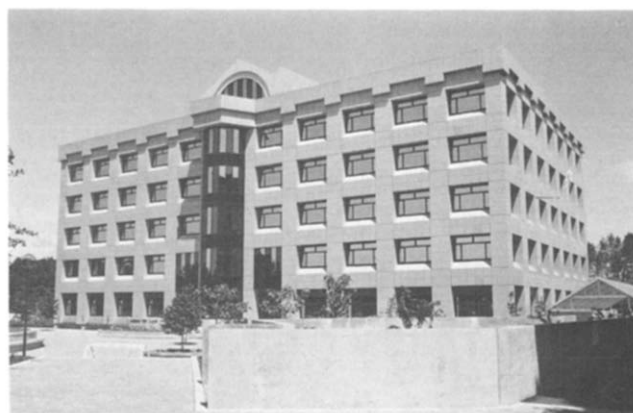
Fig. 6. Recent five-storey office building.
