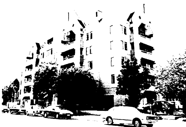
Fig. 7. Six-storey reinforced concrete hostel building.
